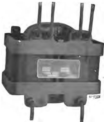
FIG. 181. 200-watt potential transformer. Wagner Electric Co.
